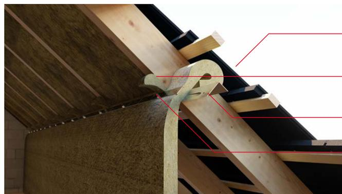
Allow sufficient material to pack and stitch Fire Barrier between rafters as shown
